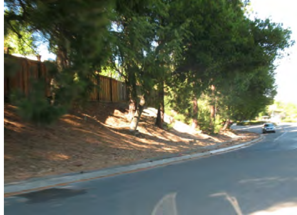
Figure 3-28 Missing Sidewalk in West Pleasant Hill
