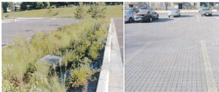
Examples of Rain Garden (left) and Permeable Pavers (right)
